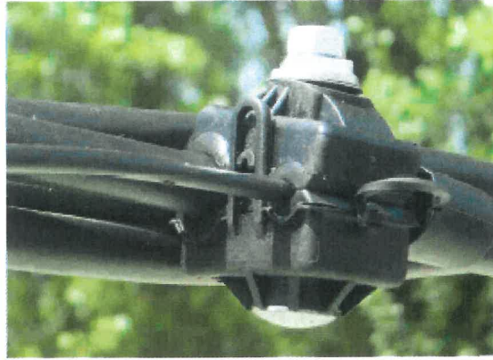
Figure 30: LV insulation piercing connector (IPC)
